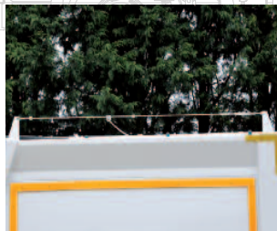
Roof Mounted Fall Prevention Safety System
